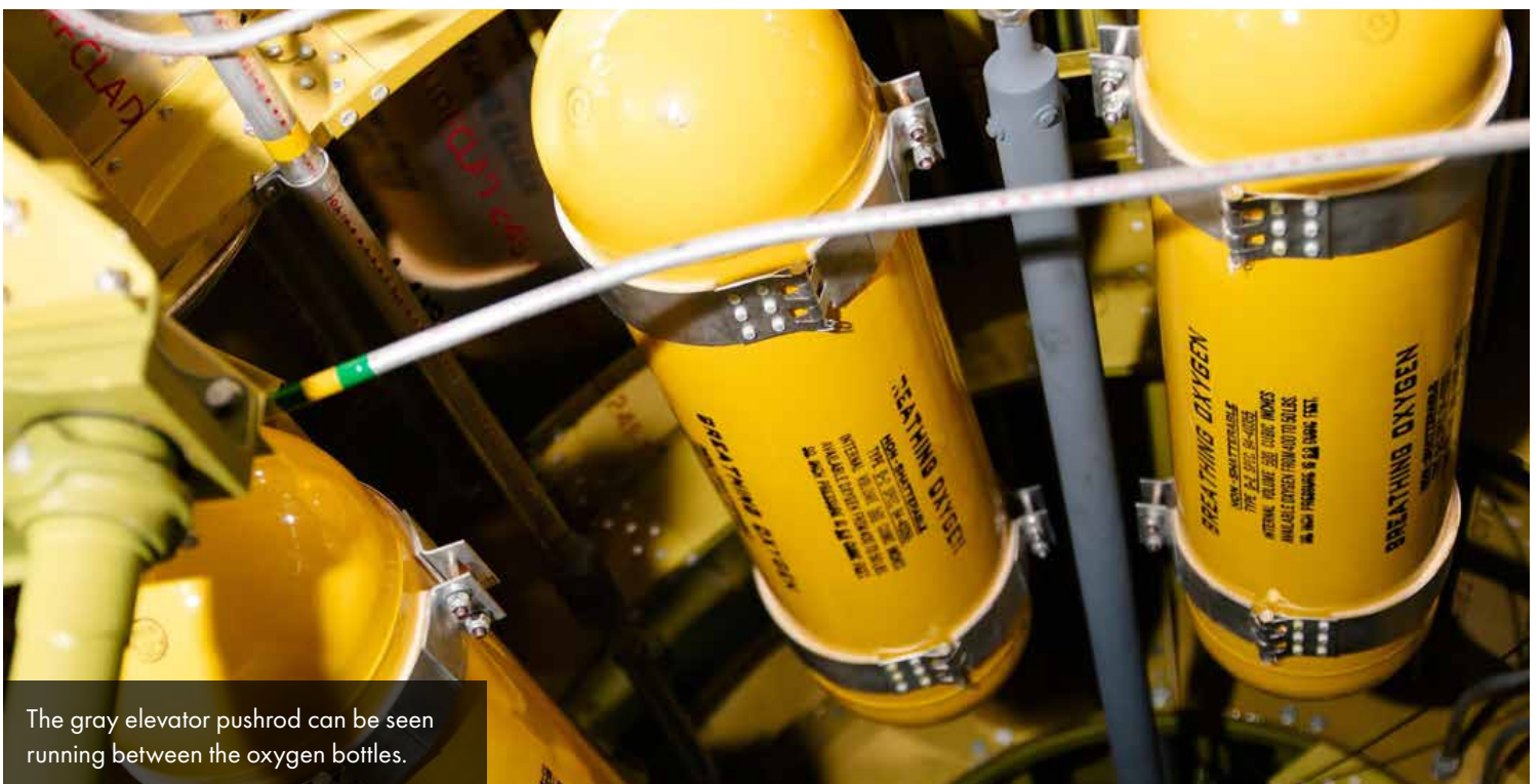
The oxygen supply and feed lines are completed.
