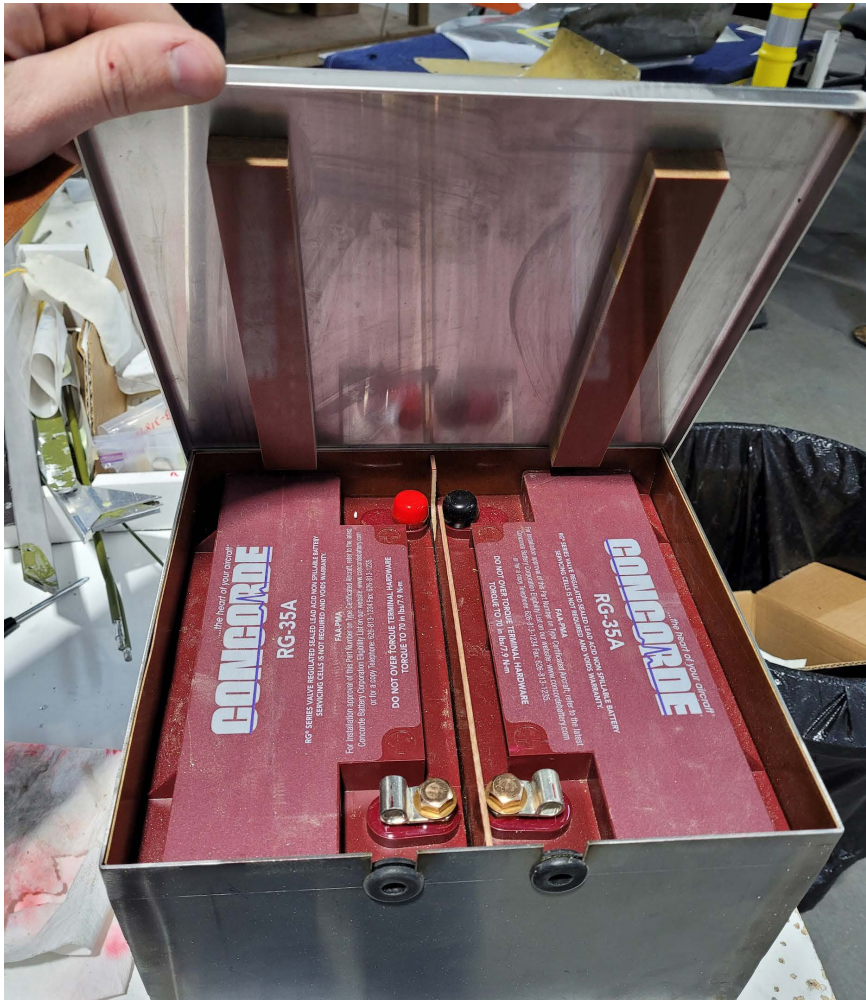
The two batteries are a tight fit in the new box.
